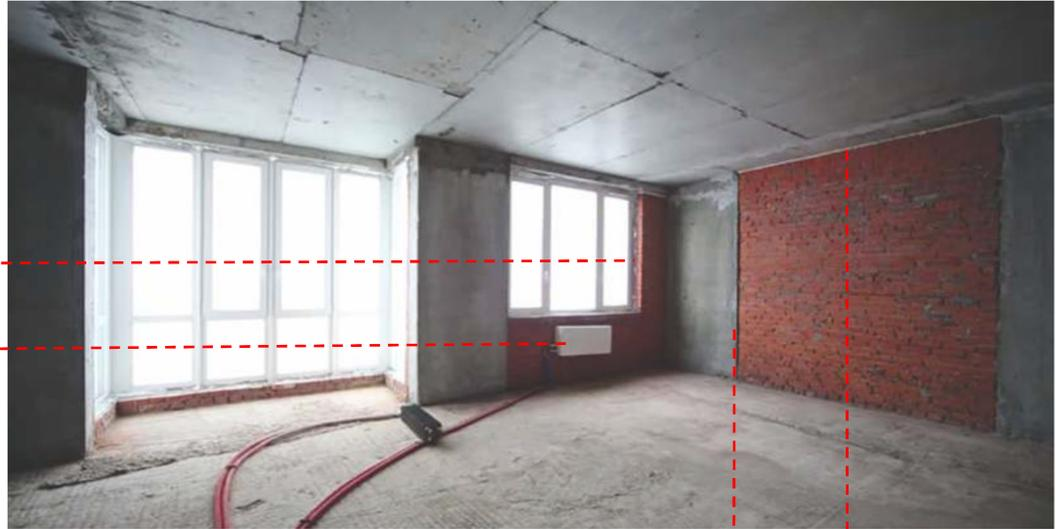
Cracks generated in between dissimilar substrates like RCC-blocks joints; brick-block joints; S\C plaster-gypsum plaster joints
